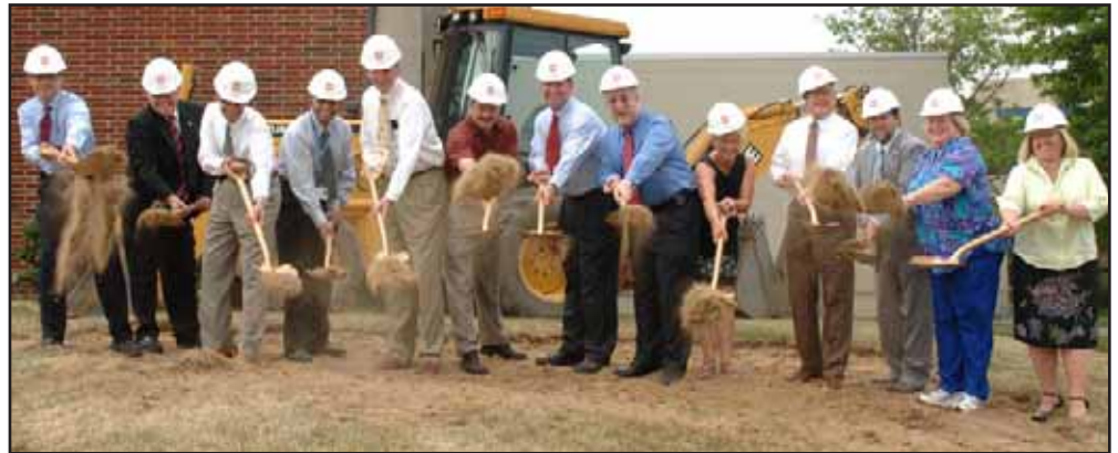
Dirt flies at the ground-breaking ceremony for the Elmer Hospital ER and MRI expansion project.
